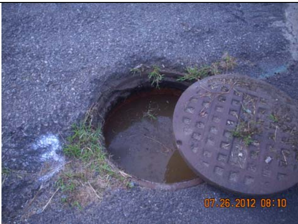
MANHOLE 4 – Abandoned Manhole (Sign Not Installed)
