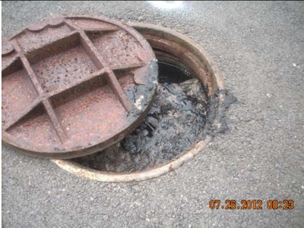
MANHOLE 5 – Abandoned Manhole (Sign Not Installed)
