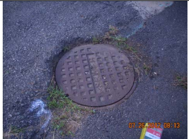
MANHOLE 4 – Abandoned Manhole (Sign Not Installed)
