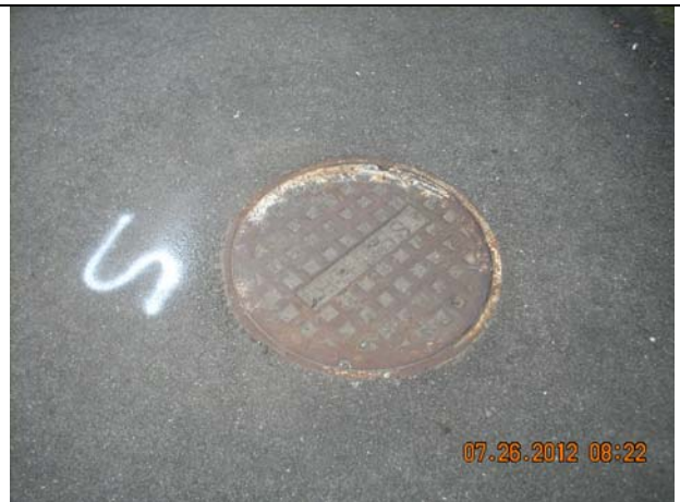
MANHOLE 5 – Abandoned Manhole (Sign Not Installed)
