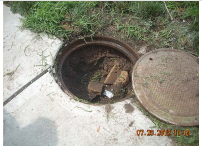
MANHOLE 10 – Abandoned Manhole (Sign Not Installed)
