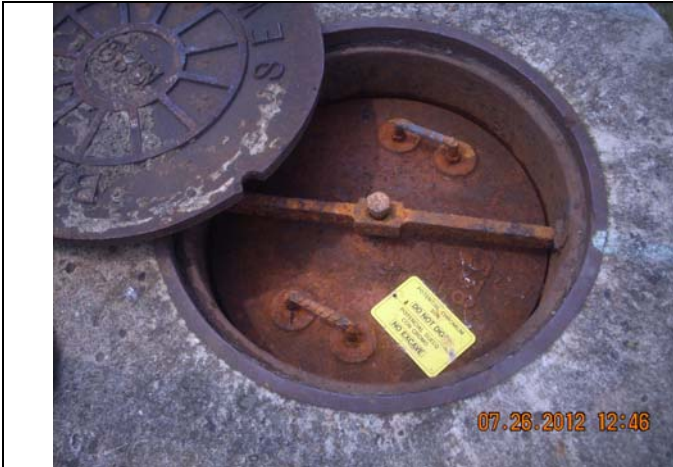
MANHOLE 11 – BMUA Cover Installation
